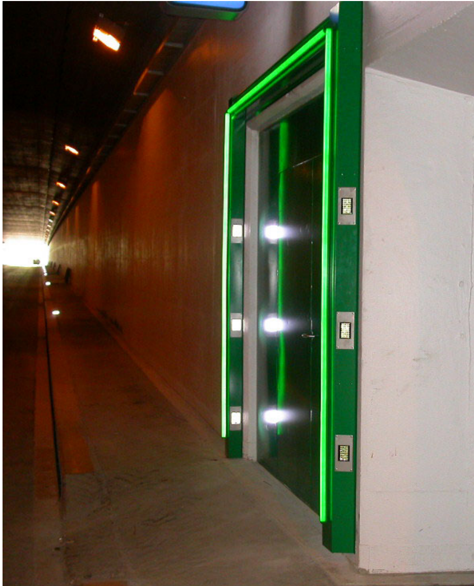
Emergency exit in road tunnel
